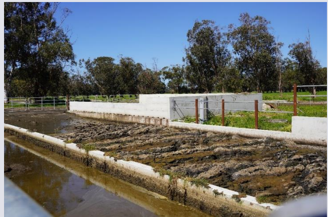
Trafficable solids trap next to effluent storage area that allows separation of solids and recollection of liquids for pond storage.
